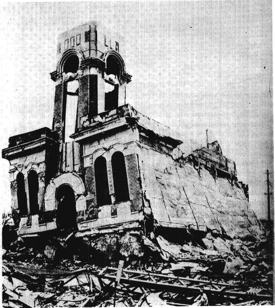
Figure 5.26. Two-story, steel-frame building with 7-inch reinforced-concrete wall panels (0.40 mile from ground zero at Hiroshima). The first story columns buckled away from ground zero dropping the second story to the ground.
