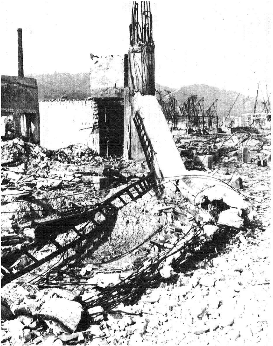
Figure 5.34b. A circular, 60 feet high, reinforced-concrete stack (0.34 mile from ground zero at Hiroshima). The failure caused by the blast wave occurred 15 feet above the base.
