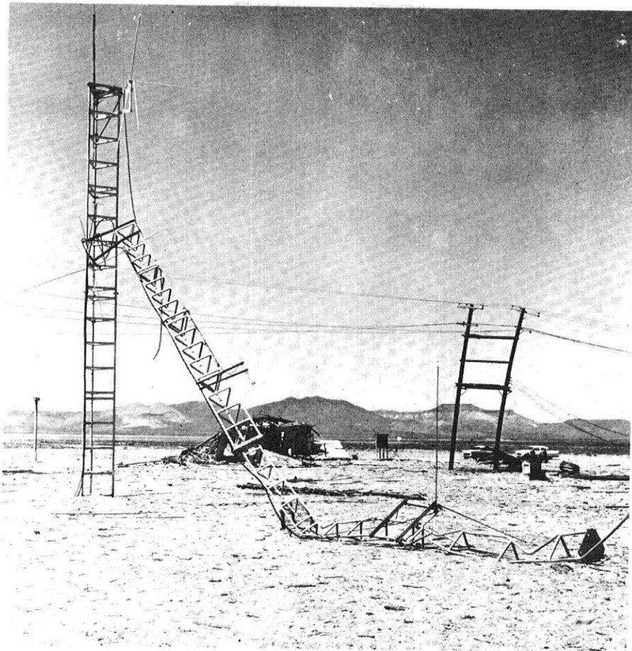
Figure 5.124. Unguyed lightweight 120-foot antenna tower (5 psi peak overpressure, 0.6 psi dynamic pressure from 30-kiloton explosion), Nevada Test Site.
