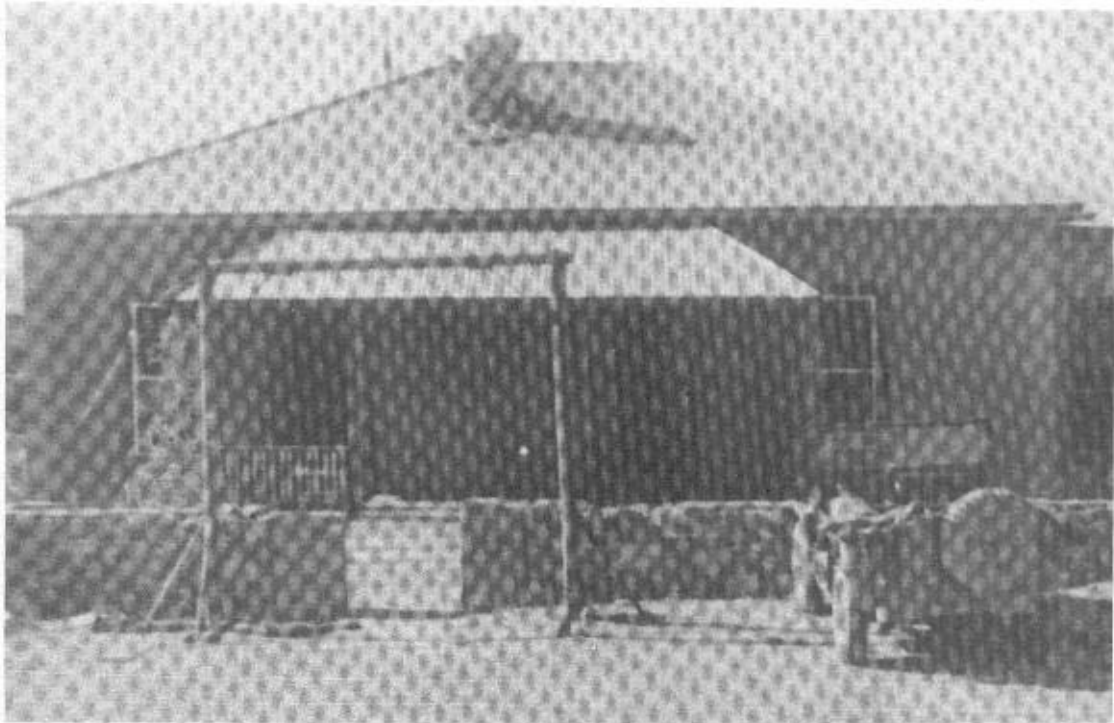
Carl Rudder's photo of the McDonald ranch house after the test.
